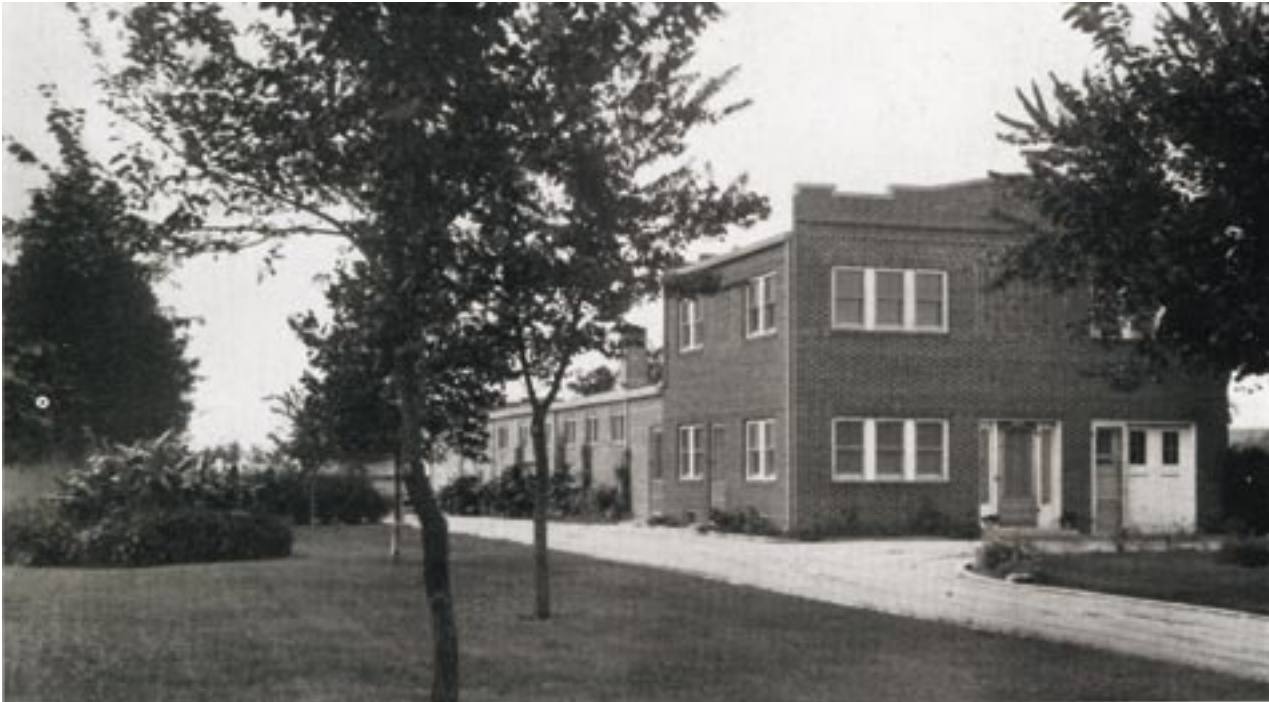
After a fire destroyed their first hatchery in Cushing, the Andersons would rebuild a new and expanded hatchery in St. Paul. It helped put the town on the map. The building still stands. Courtesy of Jane Anderson of St. Paul.
