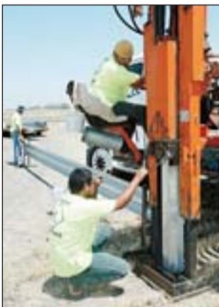
Above: Emilio Leija and other employees of Garcia-Chicoine Enterprise make a curve in guardrails being installed along the future track at Motorsport Park Hastings on Friday. Right: Jose Luis Gomez, back, and David Solano use machinery to hammer guardrail posts into the ground Friday at Motorsport Park Hastings.
